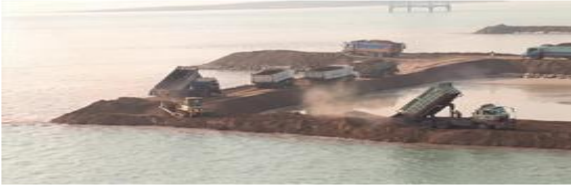
Fig 6. Construction of Coffe-Dam
