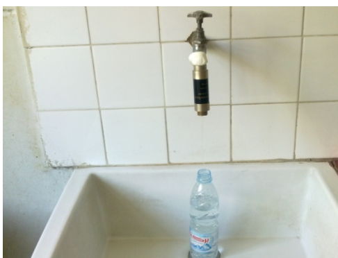
Fig. 1: The magnetic apparatus in the tap water
